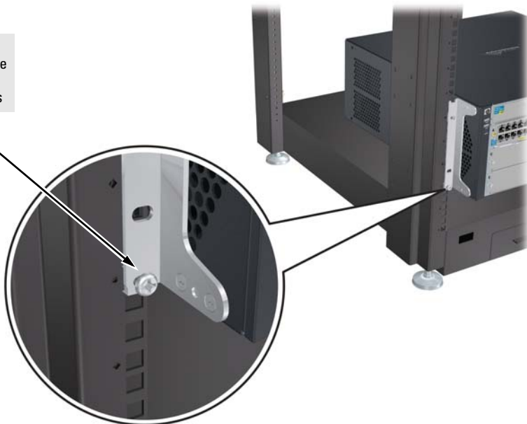
Figure 2-9. Notches in Bracket Being Installed
